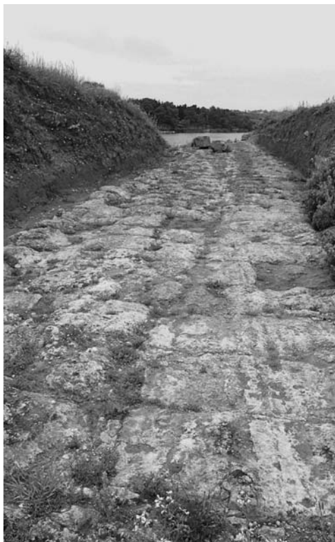
43.5. Remains of the ancient Diolkos road that allowed ships and their cargo to be dragged across the Isthmus of Corinth.
