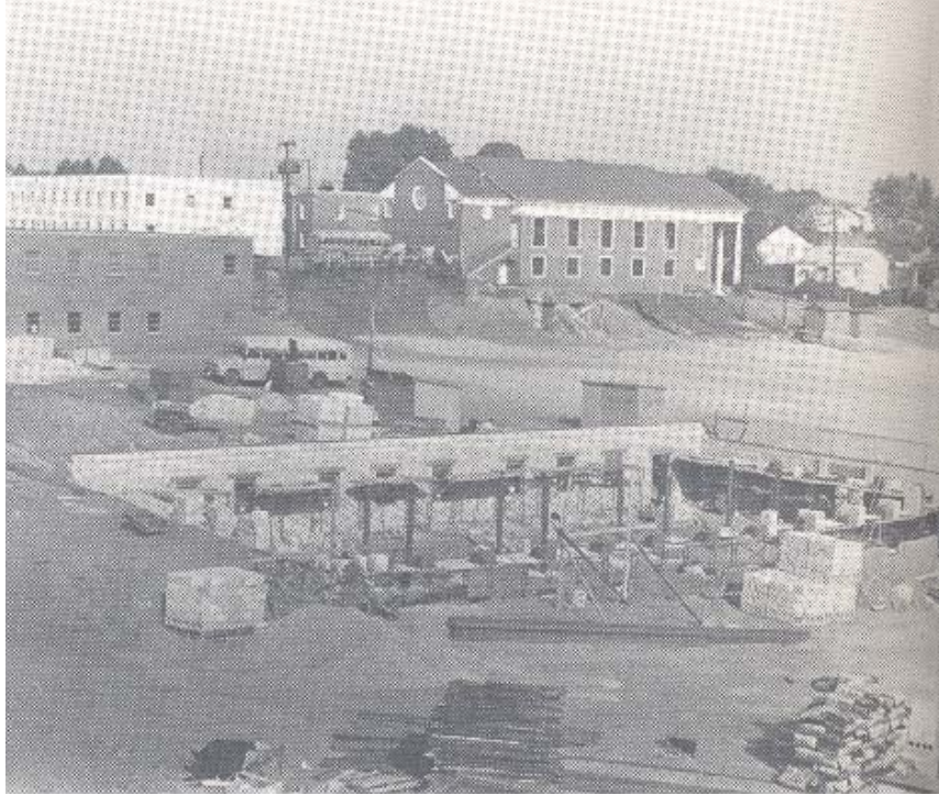
The Educational Building and new sanctuary under construction.
