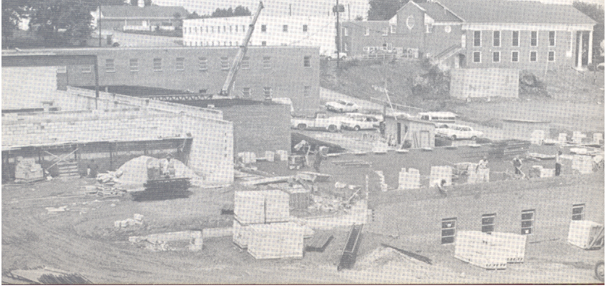
The Education Building goes up rapidly after the groundbreaking.
